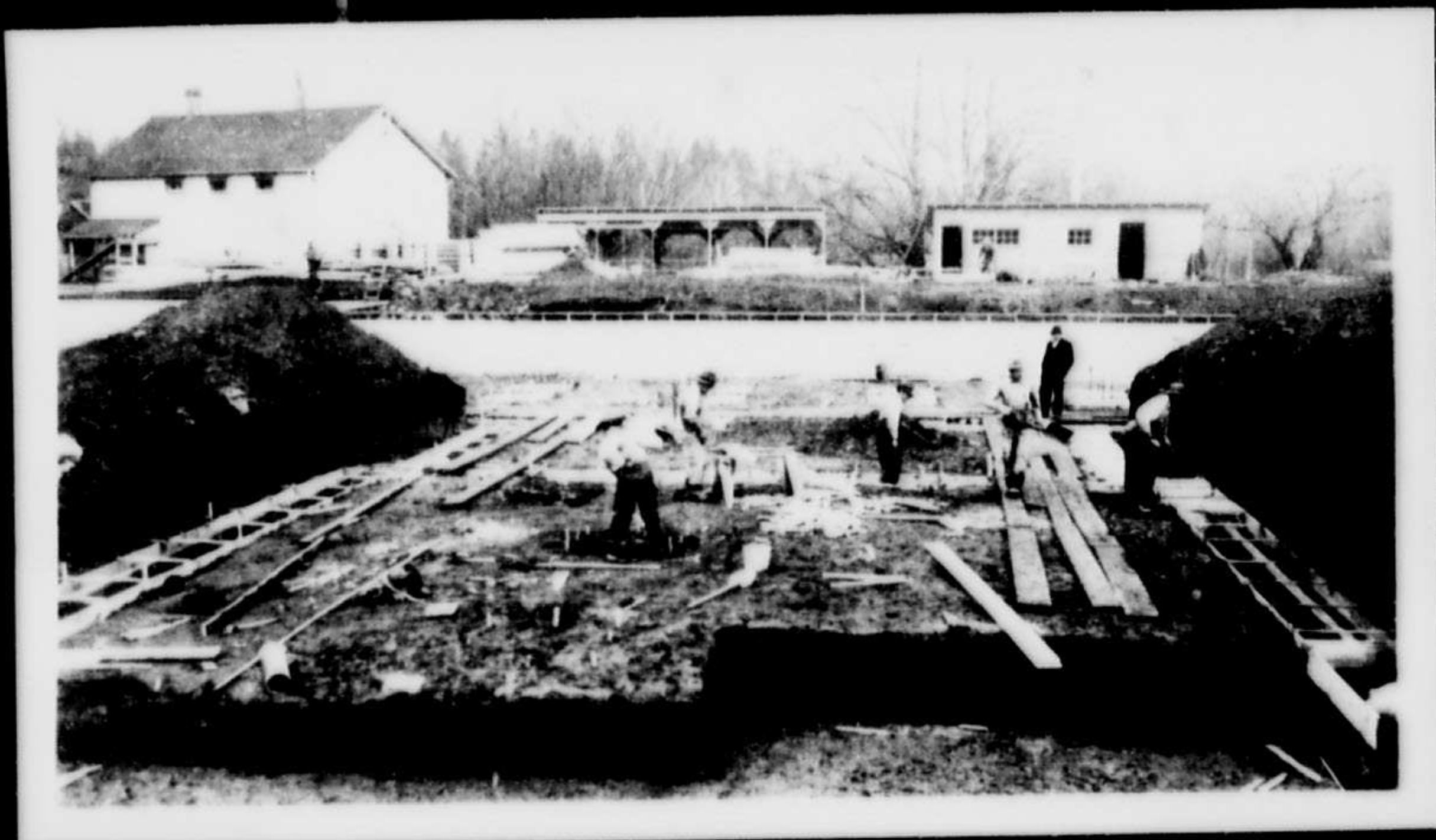
Indian Residential School, Alberni, B.C. Nov. 28/39. Looking south. Boiler room excavation in foreground.
