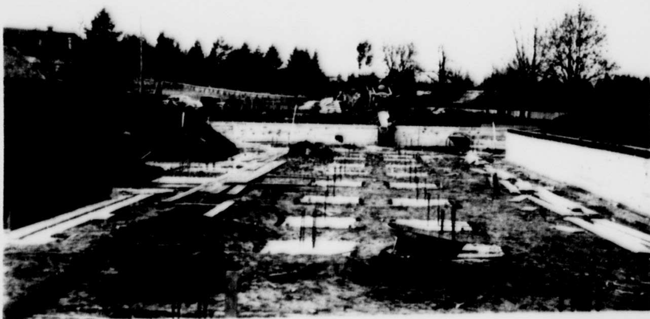
Looking East along centre line of centre wing. Indian Residential School, Alberni, B.C., Nov. 28, 1939.
