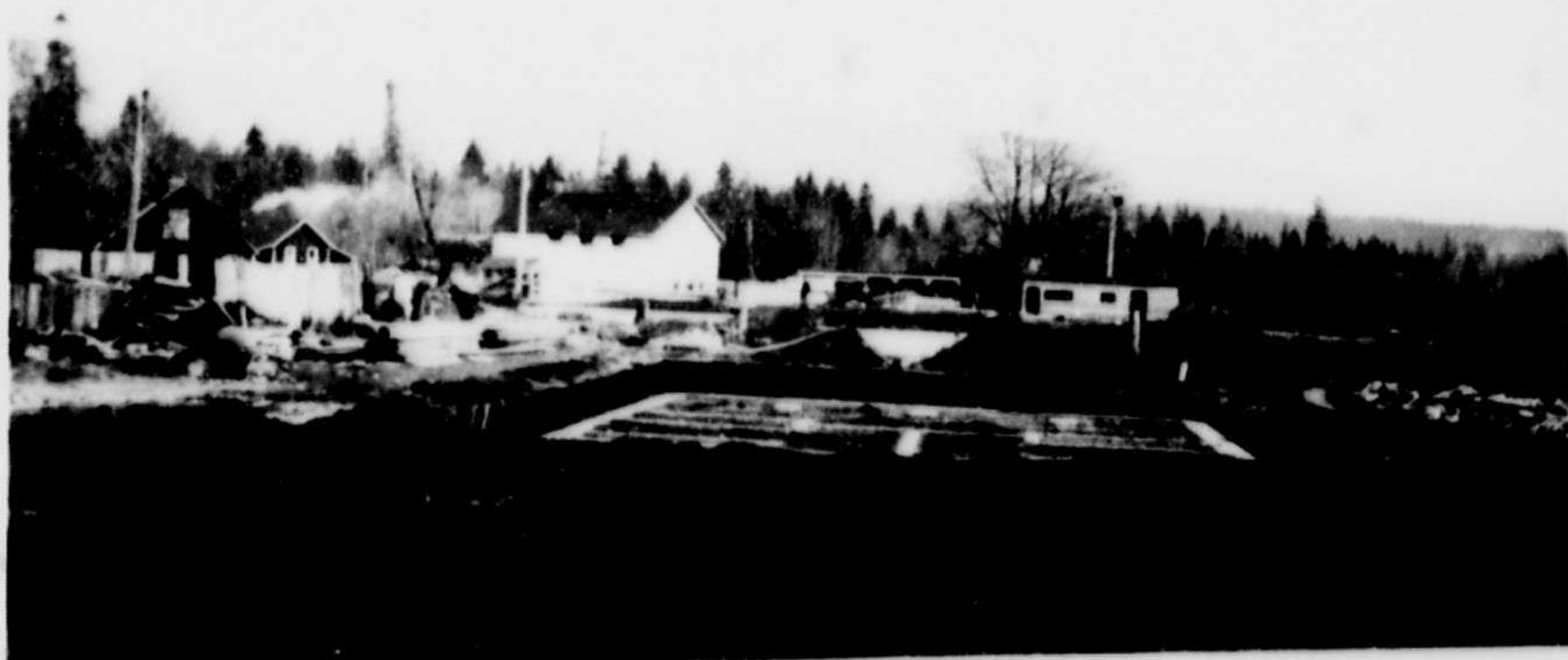
Indian Residential School, Alberni, B.C. Nov. 28/39. General view looking south. Classroom bldg. footings in foreground.
