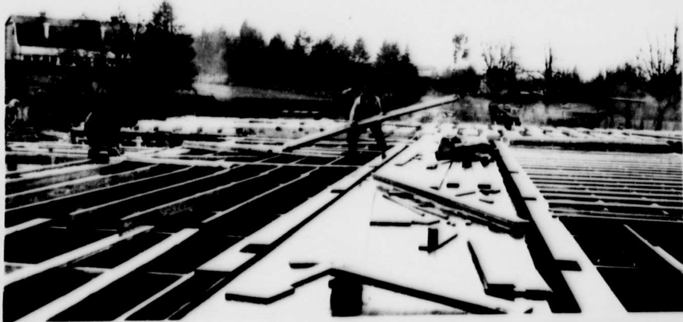
Indian Residential School, Alberni, B.C. Dec. 16/39. Looking East, 1st floor framing.
