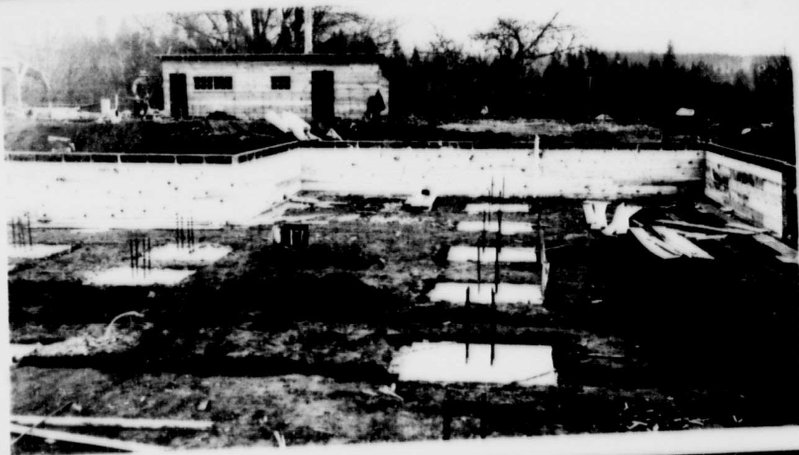
Indian Residential School, Alberni, B.C., Nov. 28/39. Looking South on centre line of building. Wall and column footings in place.
