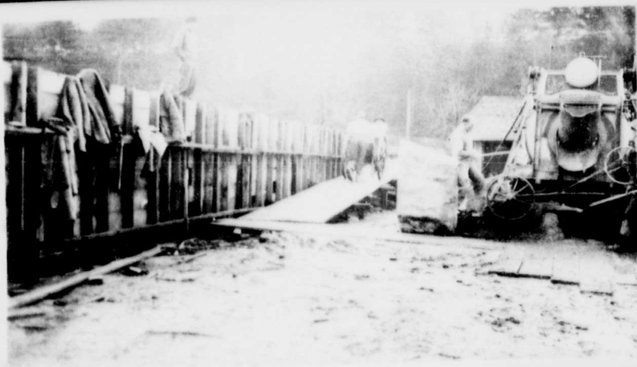
Indian Residential School, Alberni, B.C. Jan. 10/40. Concrete mixer and ramp.
