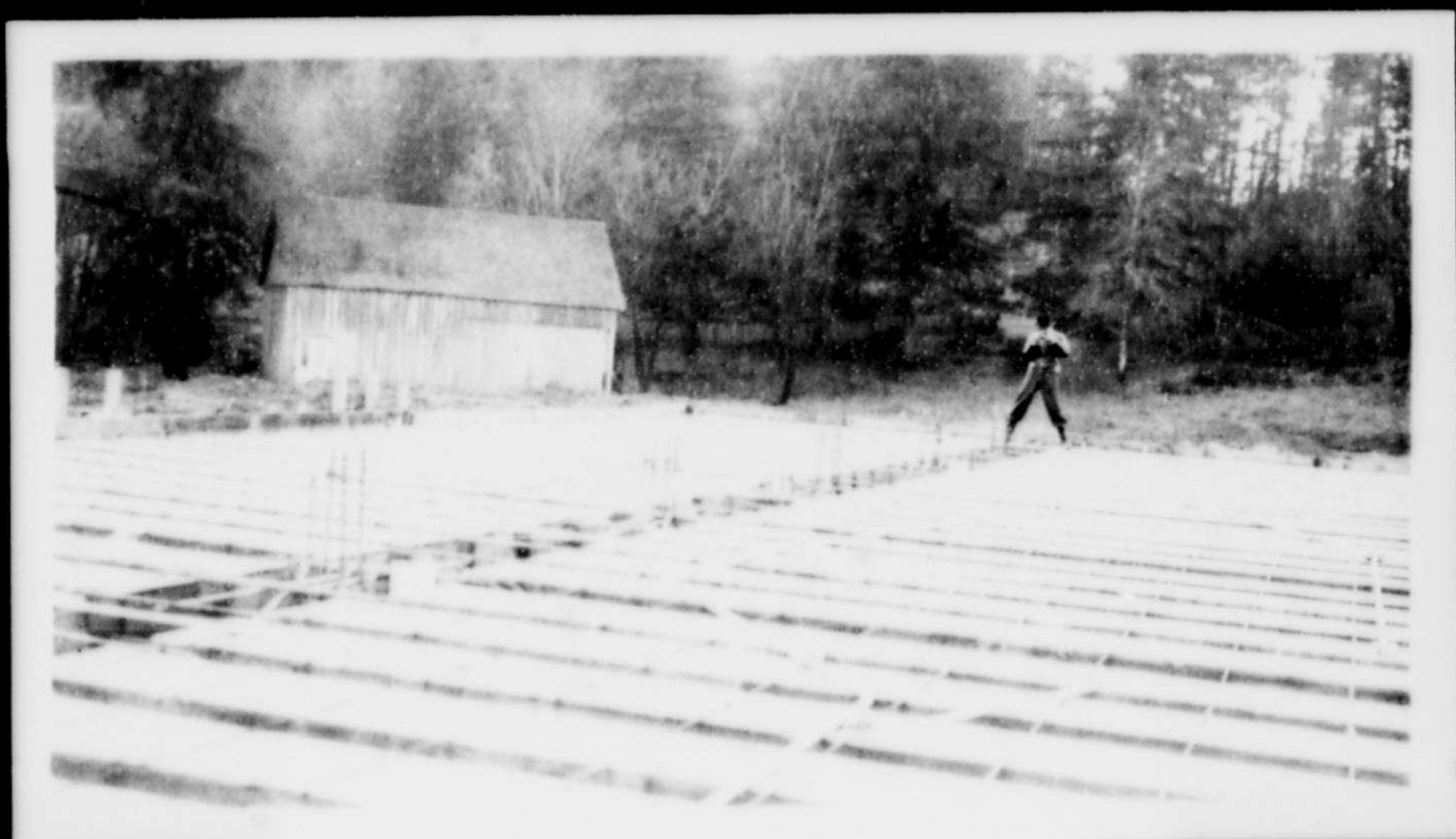
Indian Residential School, Alberni, B.C. Jan. 10/40 1st floor slab west wing ready for concrete.
